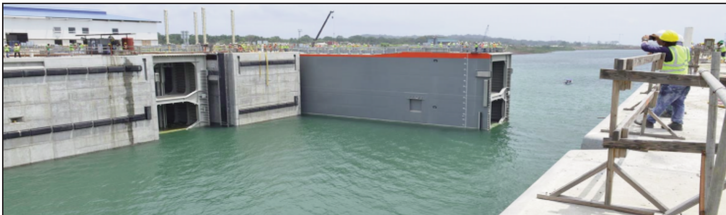
Sliding gate in the testing process. This new system does not use the "miter" type gates as used in the existing canal and most of the other river and canal locks in the U.S. of which we are most familiar.
