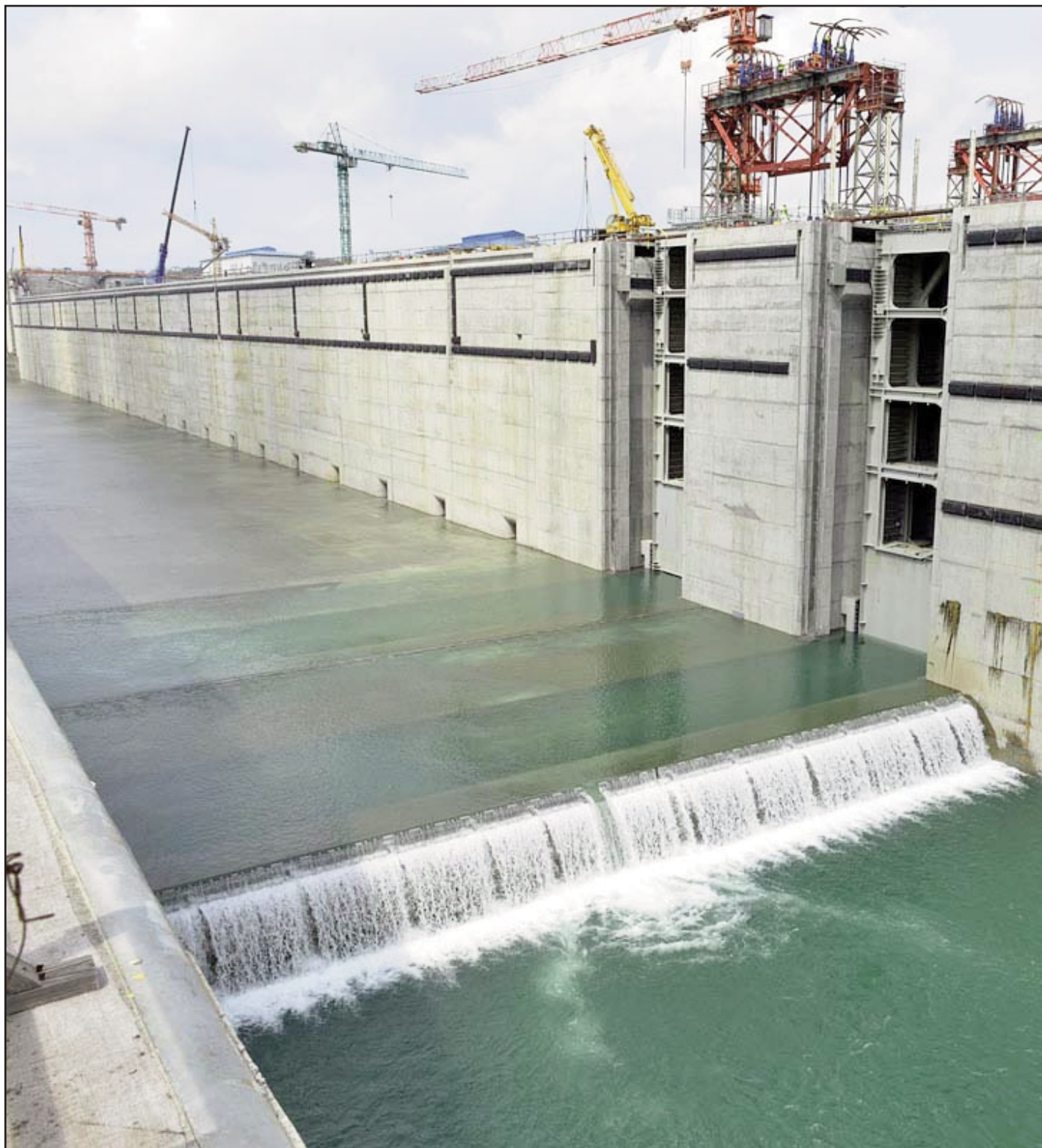
Lock chamber being filled with water from Gatun Lake
