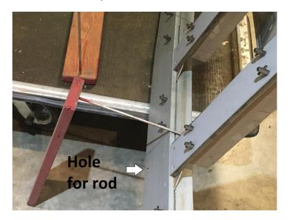
Note the reddish board with the rod. The board lays on the pond perimeter wall and the rod extended down through the small holes in the dock. We could not use the boards on the sidewalk next to the pond wall as they would be a tripping hazard, but we thought a rod through the holes in the dock directly into the pond bottom would work well and allow for the dock to move up and down with the water level.
